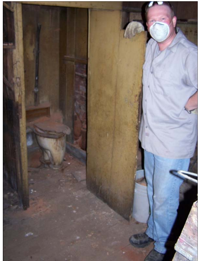
Volunteer Tom Nance with the newly accessible historic toilet in the Wah Chong Tai basement.
