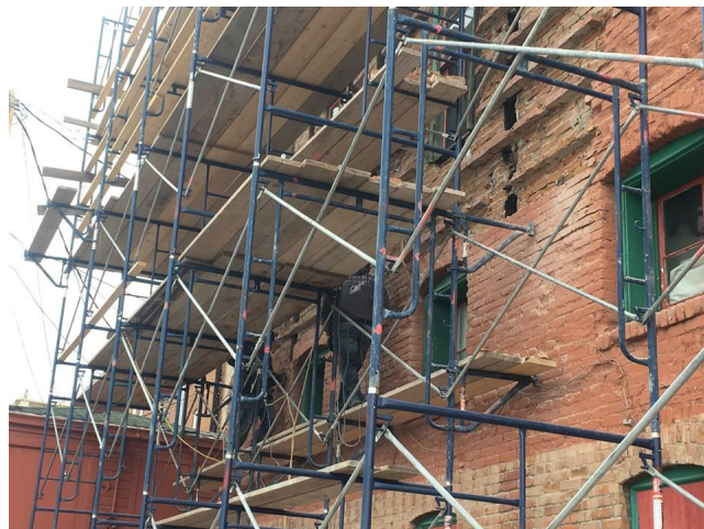
Scaffolding, west wall rebuild
