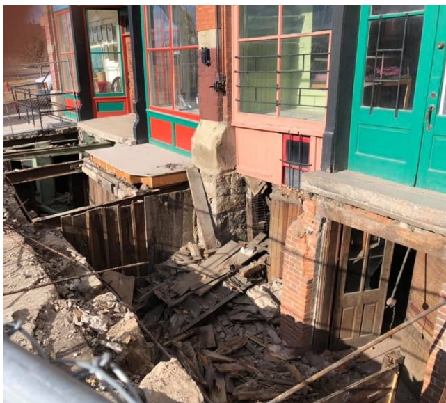
Vaulted sidewalk repair underway
