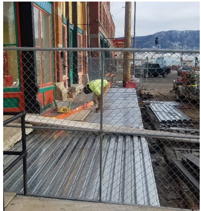
Vaulted sidewalk during reconstruction
