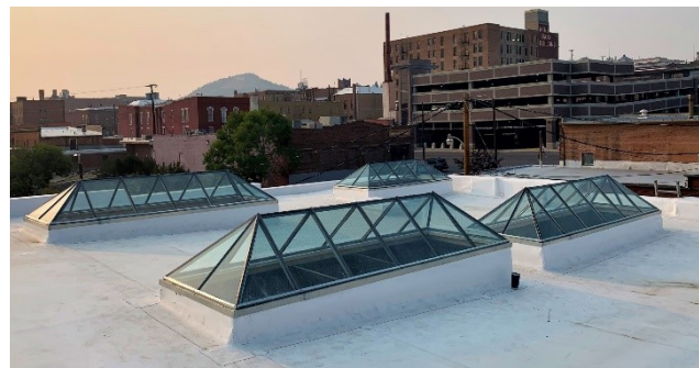
New skylights above Mai Wah Noodle Parlor
