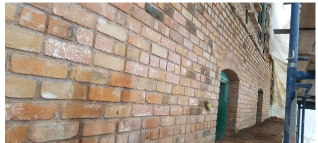
Section of west wall after reconstruction
