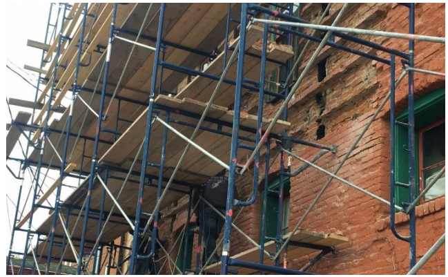
West wall during reconstruction
